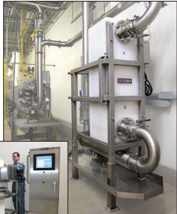
BioIonix 650 gpm installation Kidron, Ohio
